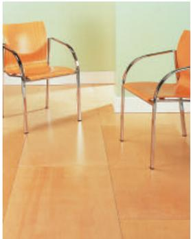
Specialist plywoods, such as Schauman Birchfloor (*see later for stockists*), provide attractive, structural and hardwearing flooring for both commercial and domestic applications. They can be laid onto a variety of surfaces, like joists or concrete, provided correct procedures are followed.
