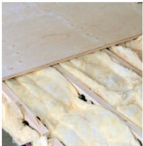
Plywood panels are fixed in much the same way as solid timber flooring:
