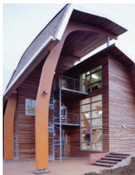
Beams or columns made from layers of parallel Pine or Spruce lamellas, cut following the grain and glued together.
