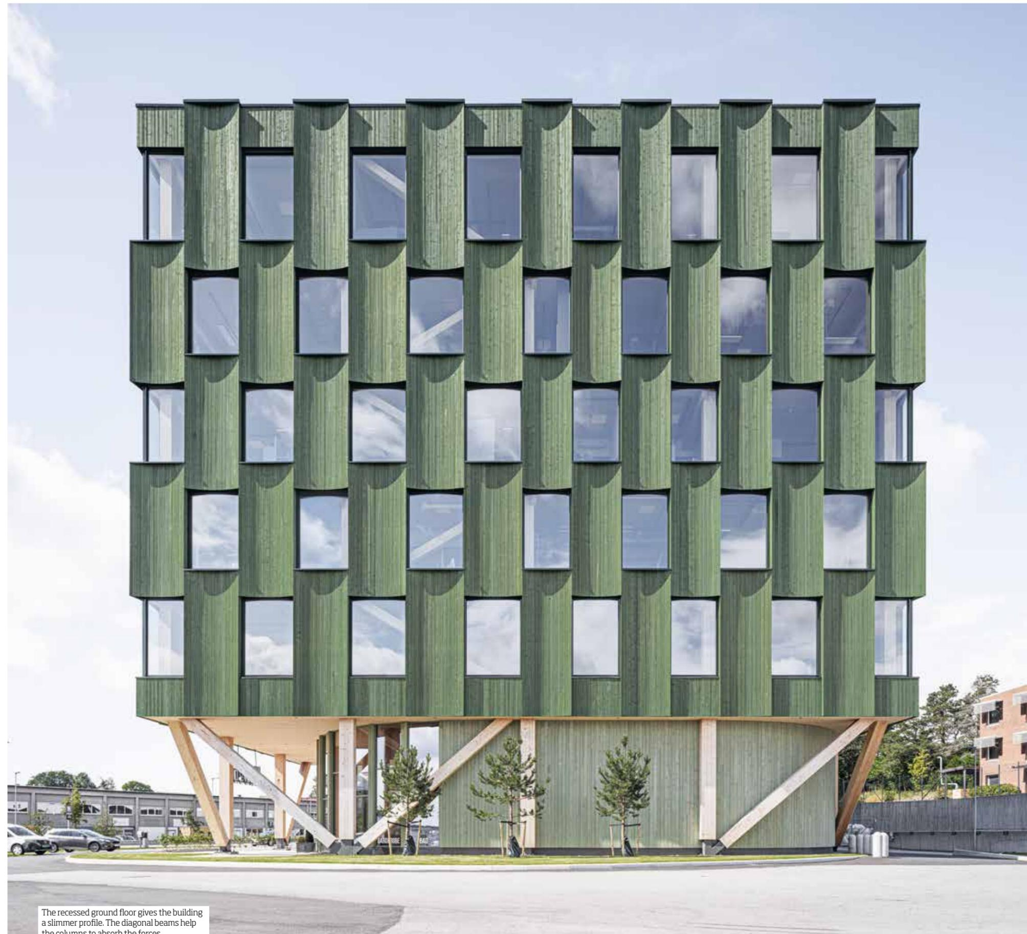
The recessed ground floor gives the building a slimmer profile. The diagonal beams help the columns to absorb the forces.
