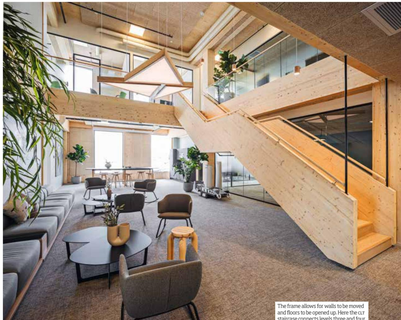
The frame allows for walls to be moved and floors to be opened up. Here the CLT staircase connects levels three and four.
