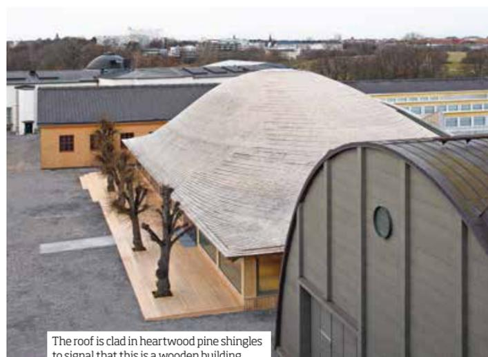
The roof is clad in heartwood pine shingles to signal that this is a wooden building.
