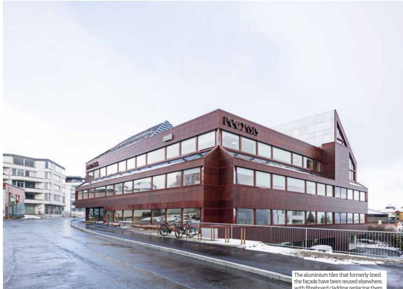
The aluminium tiles that formerly lined the façade have been reused elsewhere, with fibreboard cladding replacing them.
