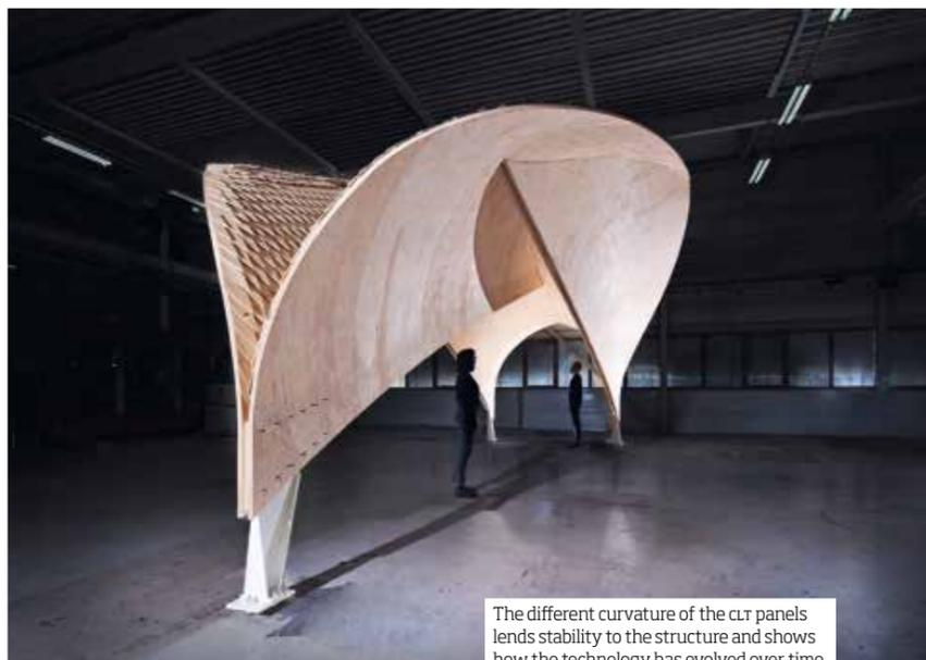
The different curvature of the CLT panels lends stability to the structure and shows how the technology has evolved over time.
