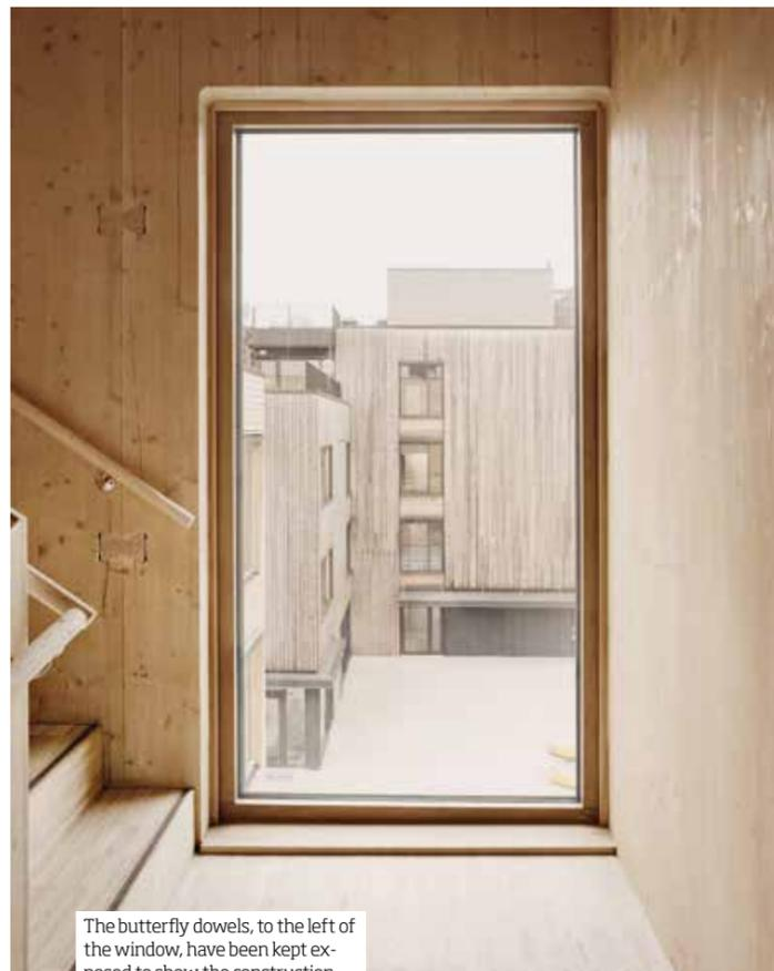
The butterfly dowels, to the left of the window, have been kept exposed to show the construction.
