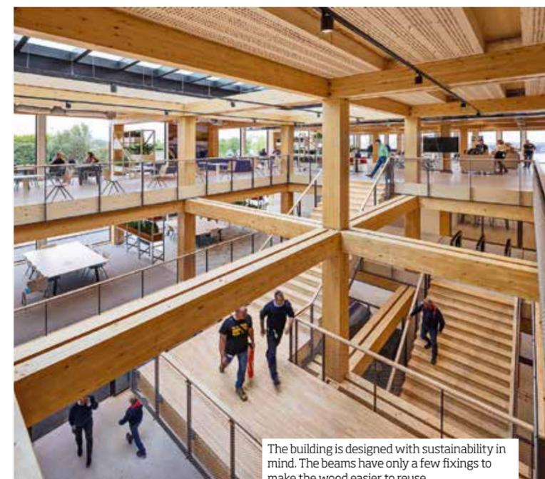
The building is designed with sustainability in mind. The beams have only a few fixings to make the wood easier to reuse.
