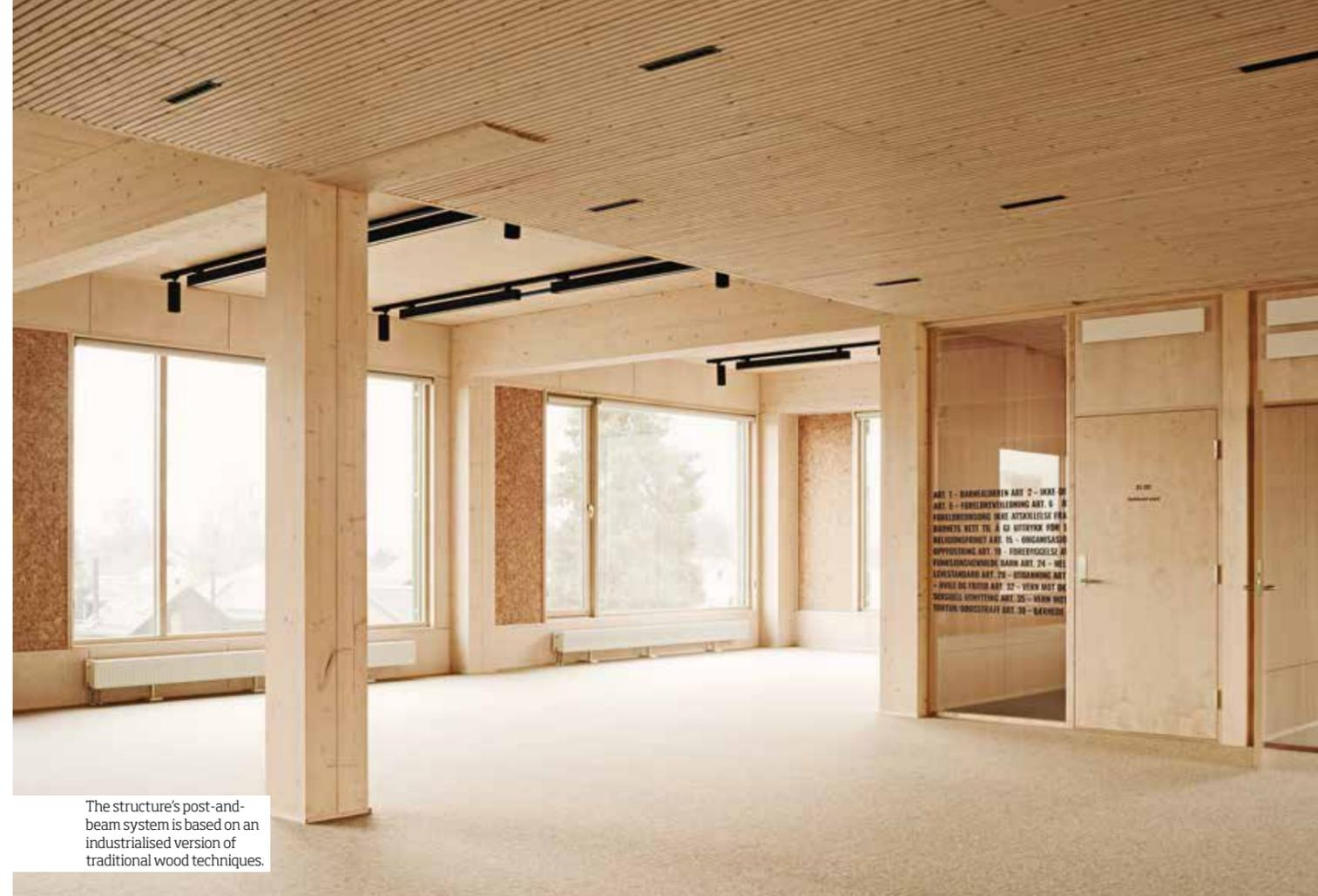
The structure's post-and-beam system is based on an industrialised version of traditional wood techniques.
