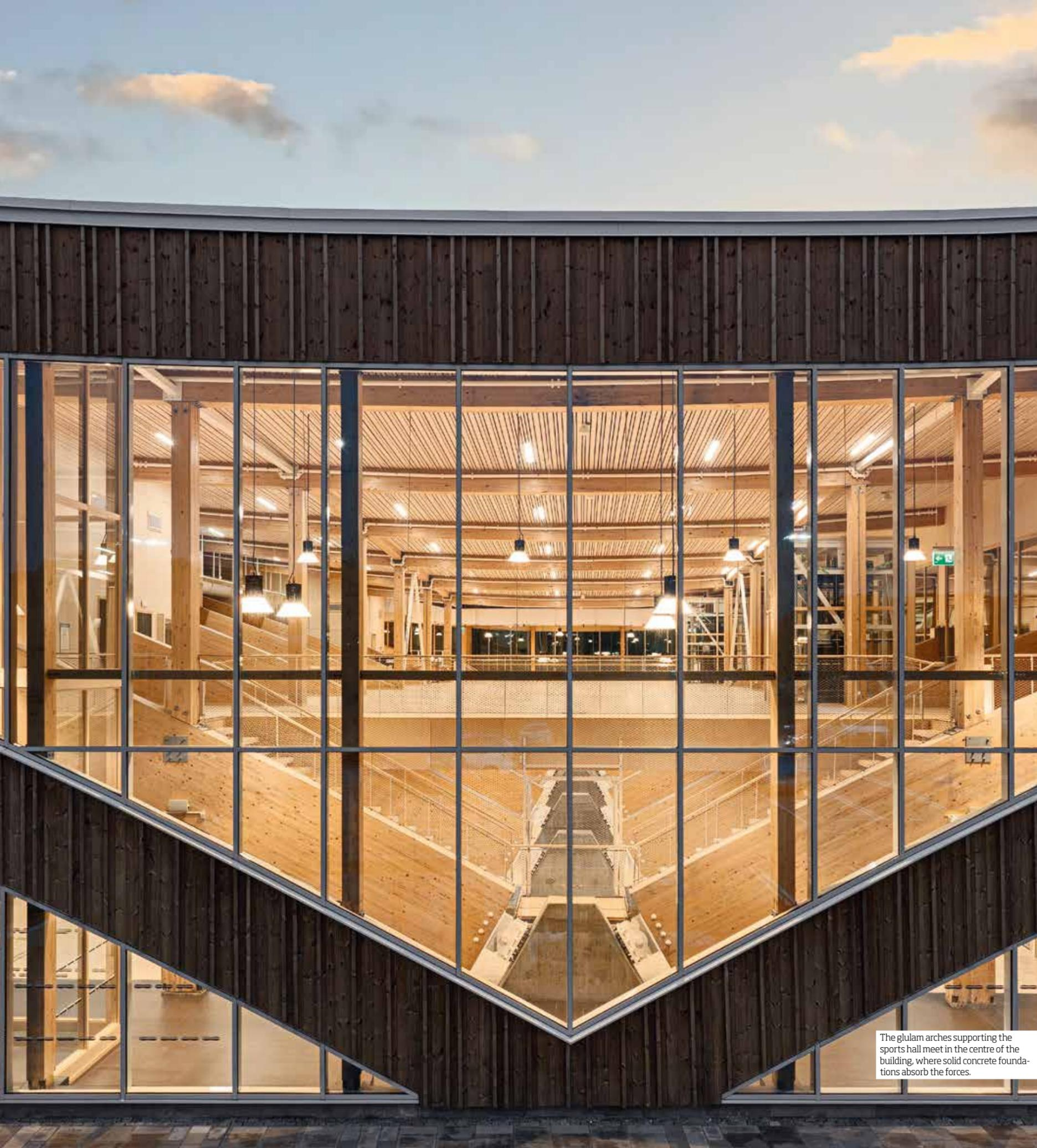
The glulam arches supporting the sports hall meet in the centre of the building, where solid concrete foundations absorb the forces.
