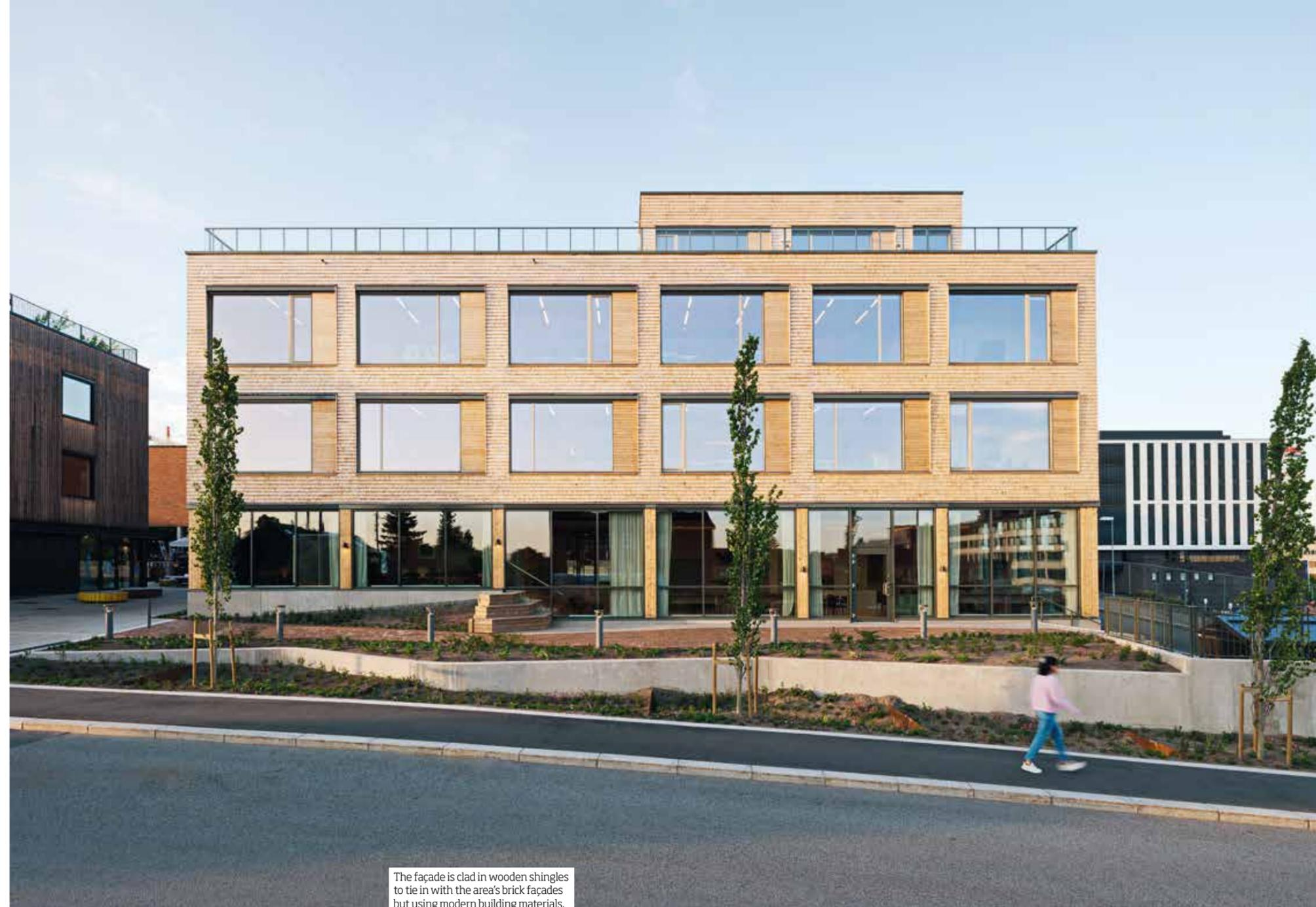
The façade is clad in wooden shingles to tie in with the area's brick façades but using modern building materials.
