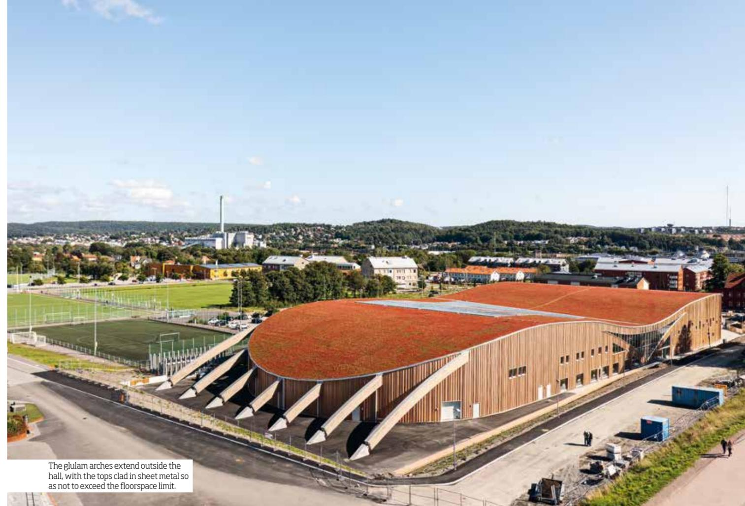
The glulam arches extend outside the hall, with the tops clad in sheet metal so as not to exceed the floorspace limit.
