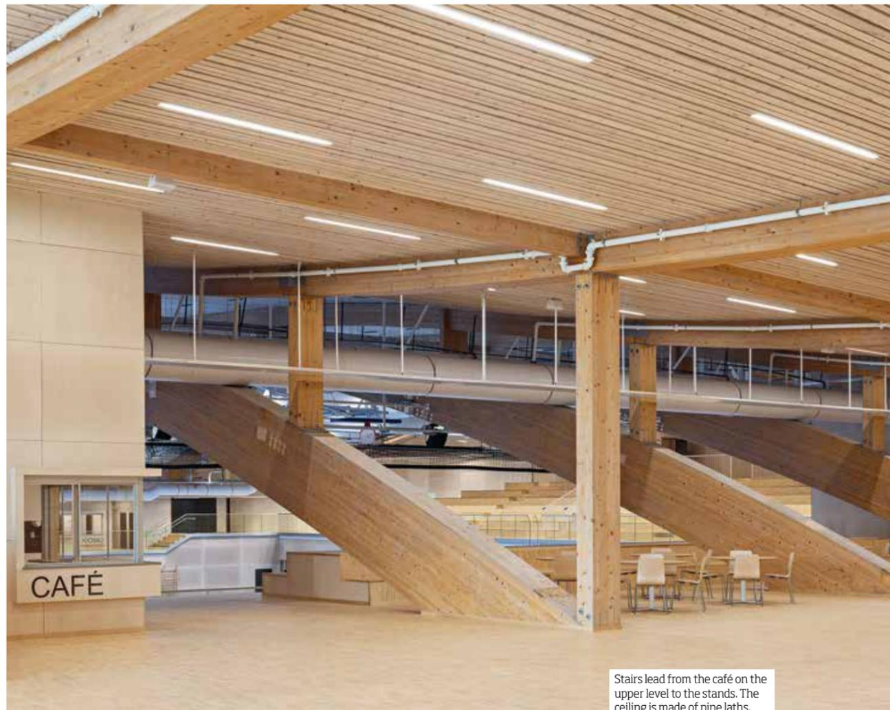
Stairs lead from the café on the upper level to the stands. The ceiling is made of pine laths.
