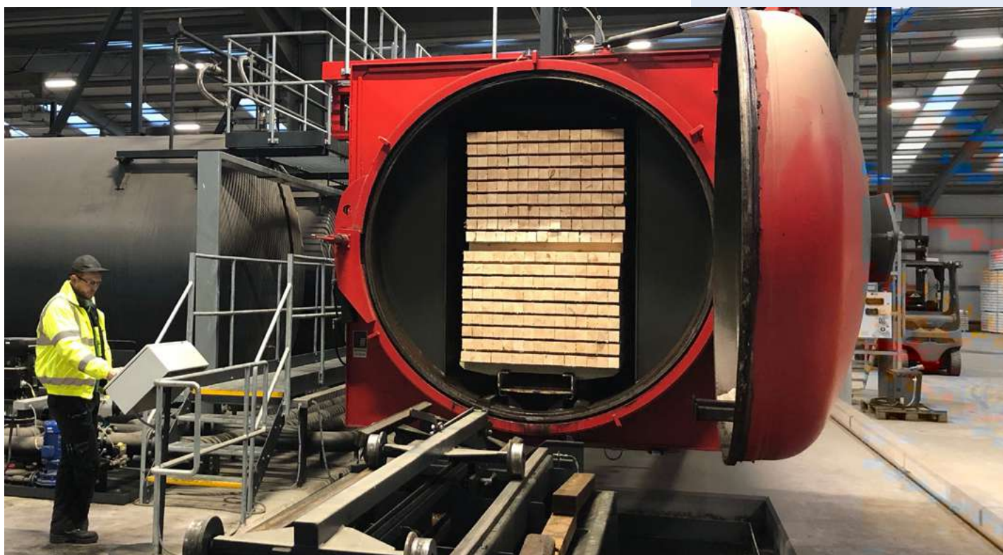
A typical wood preservative pressure treatment plant. Photo courtesy of James Jones & Sons Ltd.
