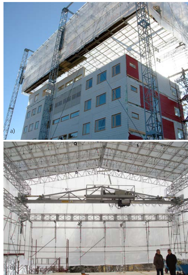
Figure 8.14 a) Movable tent over the whole building. Älvsbacka Strand, Skellefteå. b) Movable tent from the inside with integrated travelling crane.
