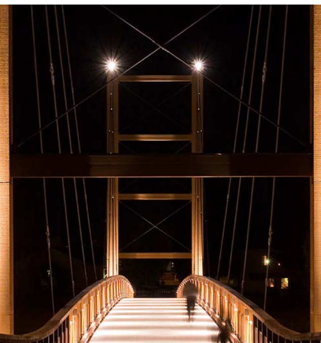
Pedestrian and bike cable-stayed bridge, Skellefteå.
