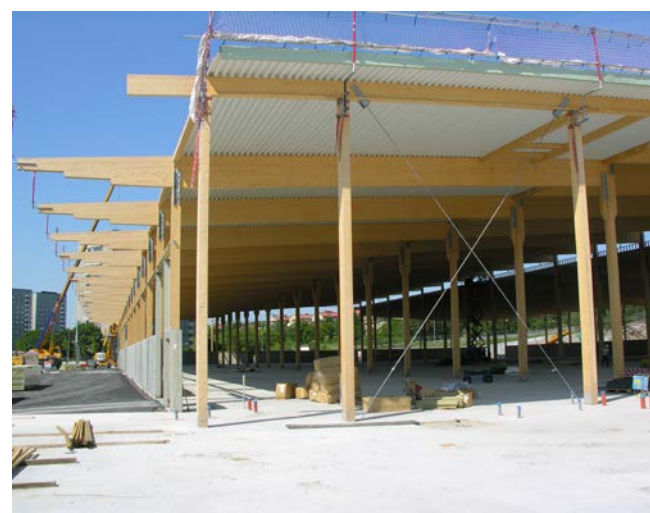
Glulam hall under construction. Permanent cross bracing at a gable wall transfers horizontal loading from stiff roof sheet to the ground
