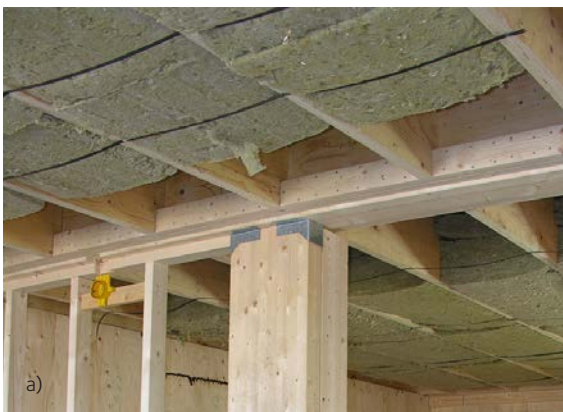
Figure 3.1 Examples of flexural members. a) External timber structure, b) floor joists.
