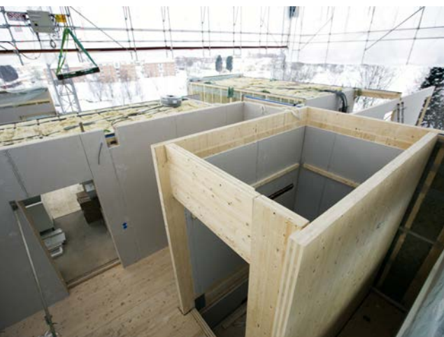
Elevator shaft of CLT.
