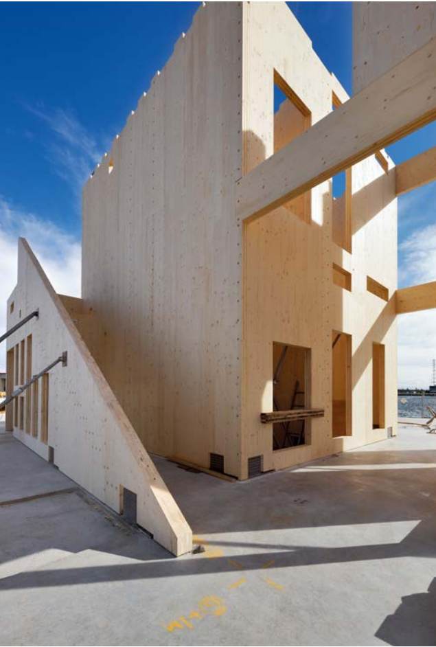
Assembly of CLT walls.
