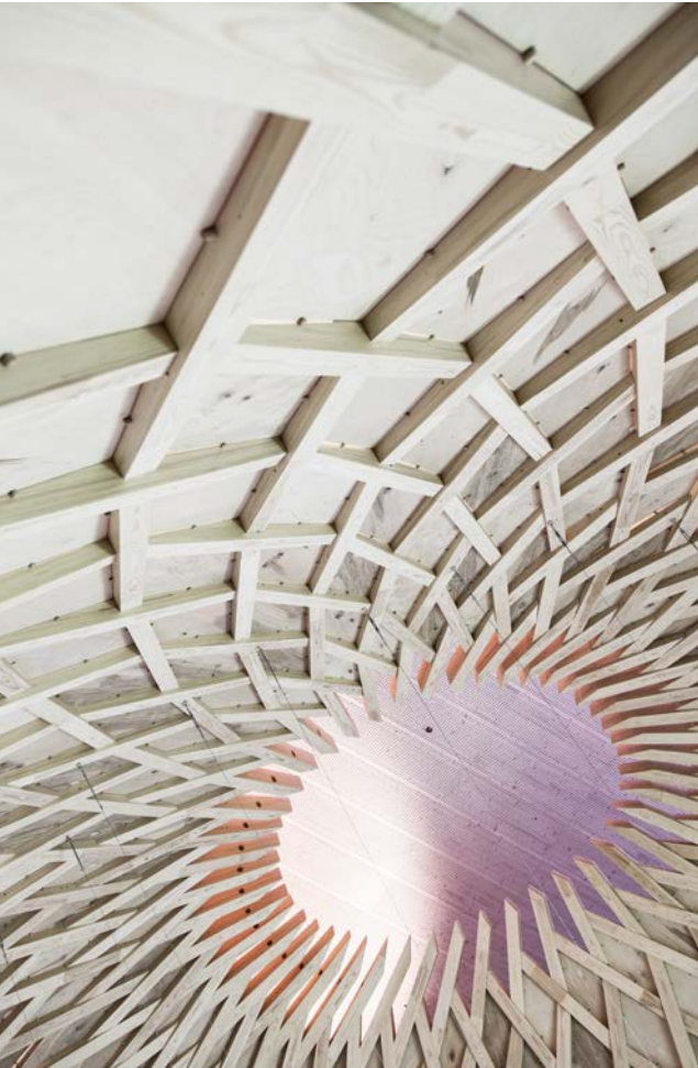
Roof made of glulam and CLT.
