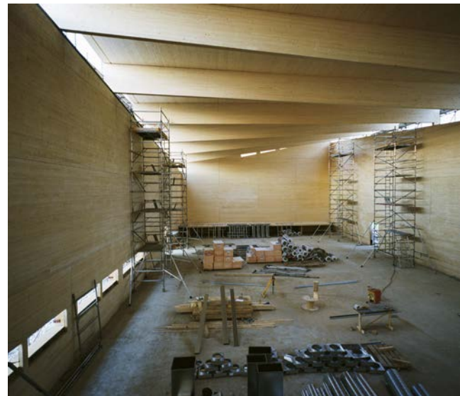
Kingsdale School sports hall, London, England.
