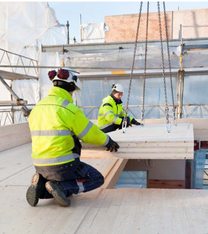
Assembly of CLT floor.
