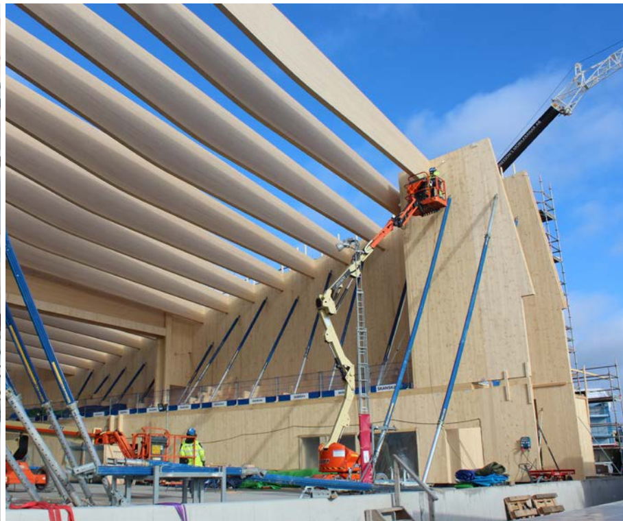
Stabilising using braces during construction.
