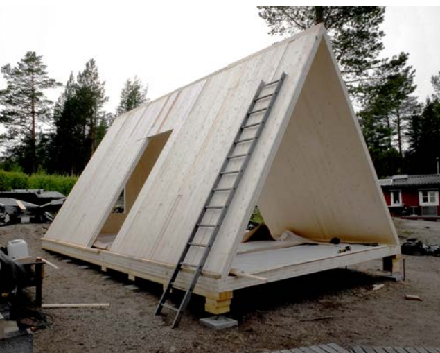
Assembly of a summer house, Skellefteå, Sweden.
