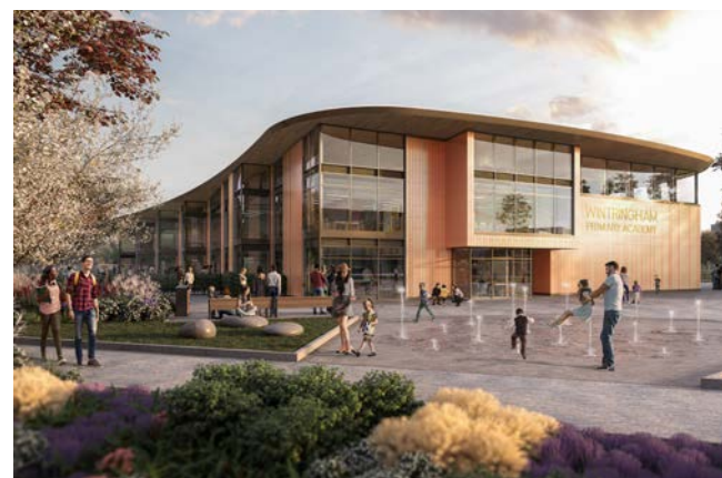
Example of a roof structure with load-bearing and stabilising CLT panels, which also contribute to a good indoor climate. Wintringham Academy, St Neots, England.
