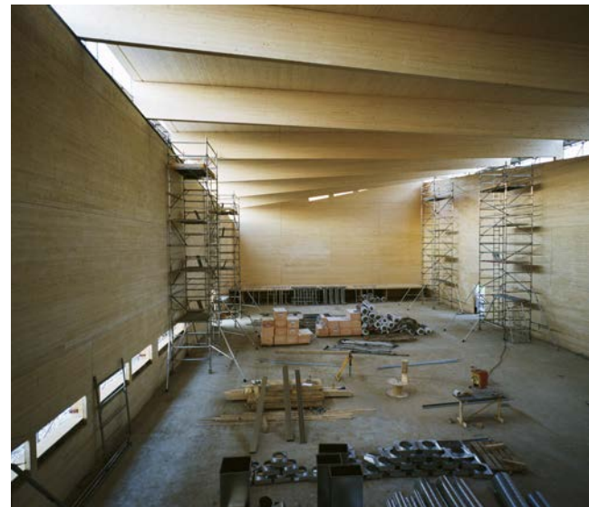
Kingsdale School sports hall, London, England.
