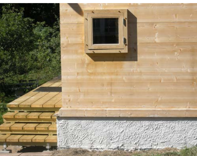
Summer house under construction, Öland, Sweden.
