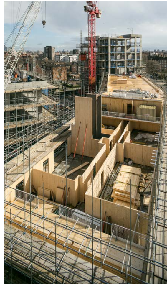
Trafalgar Place apartments, London, England.
