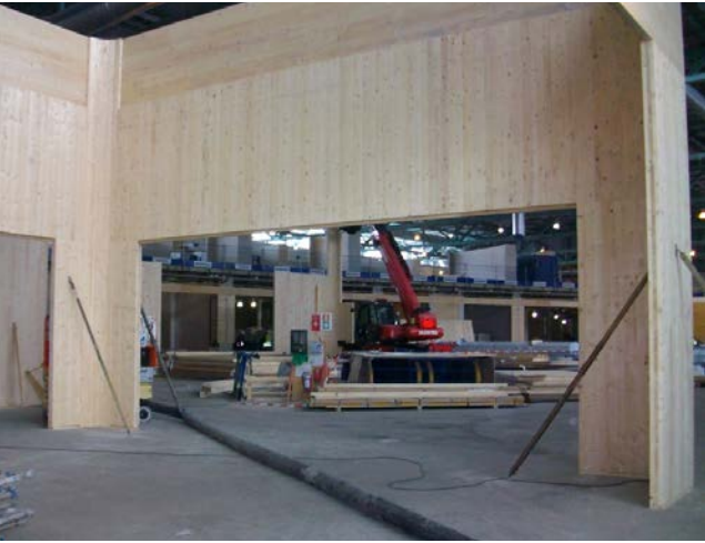
Erection of walls made of CLT, Bromma Blocks, Stockholm, Sweden.
