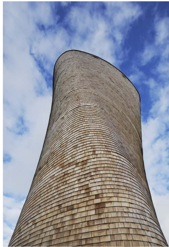
Ventilation tower with CLT frame, Stockholm, Sweden.
