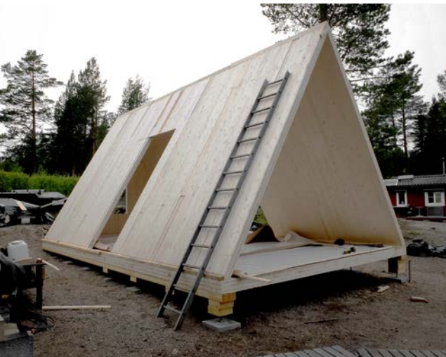
Assembly of a summer house, Skellefteå, Sweden.
