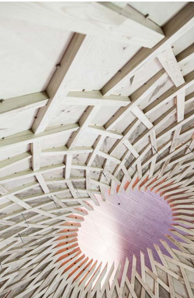
Roof made of glulam and CLT.
