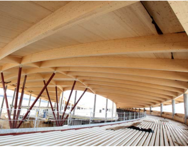
Roof made of glulam and CLT.
