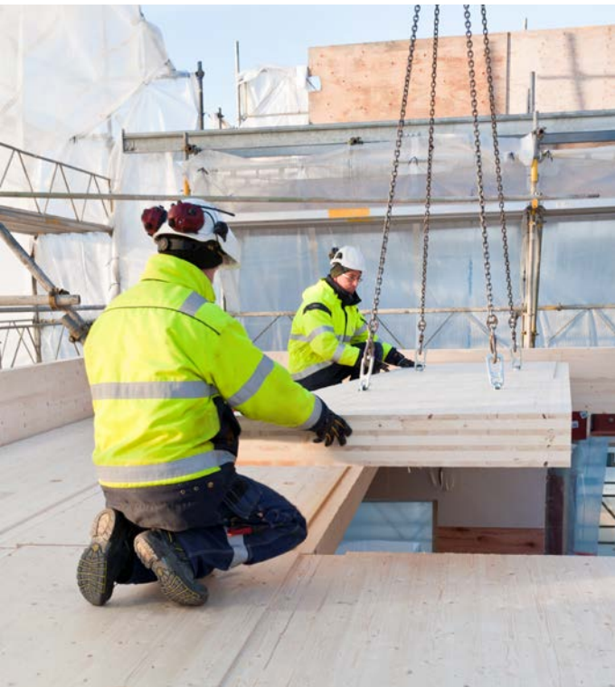
Assembly of CLT floor.
