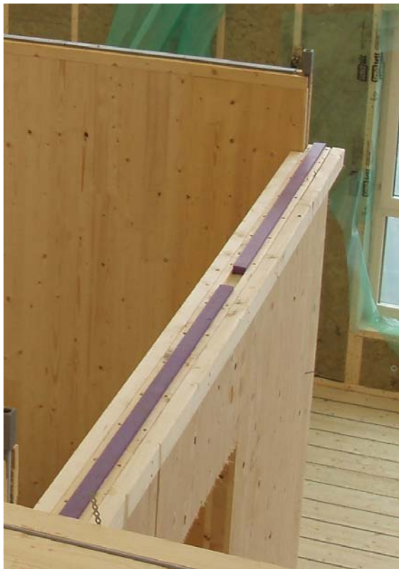
Example of vibration-damping intermediate layer.
