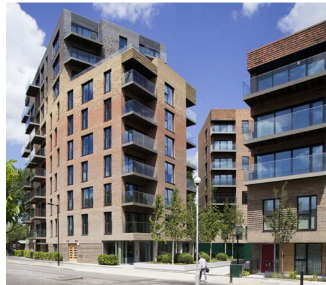
Trafalgar Place apartments, London, England.
