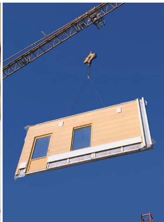
Lifting a prefabricated wall unit.
