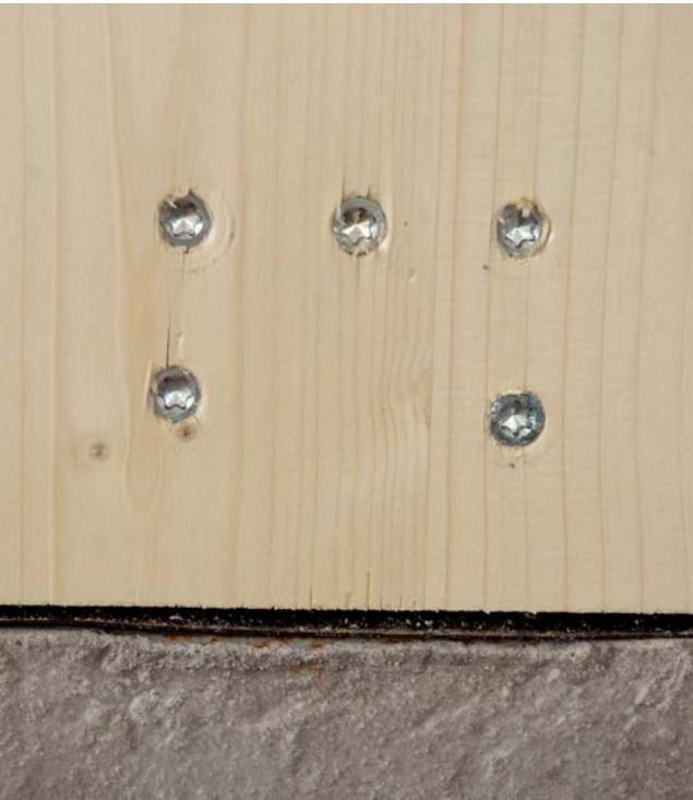
Screwed joint, CLT.
