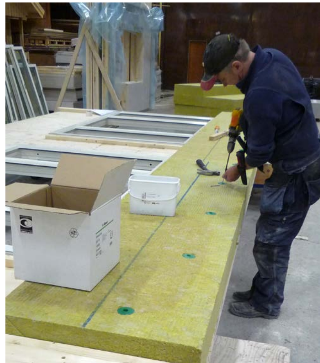
Insulation of CLT wall.
