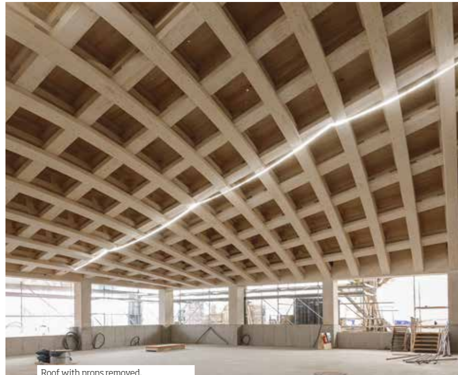
Roof with props removed.
