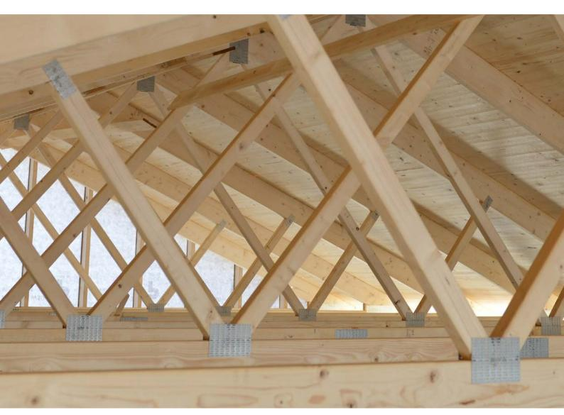
Strength graded construction timber for prefabricated roof trusses.
