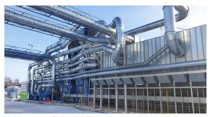
Industrial heat recovery system. To achieve maximum efficiency, careful calculation is required based on the size of the premises and the extraction requirements.
