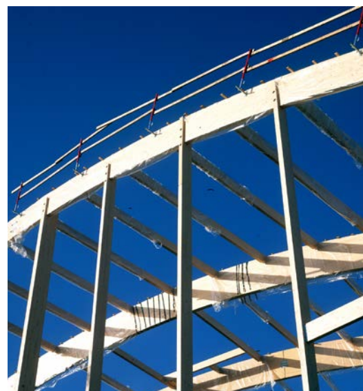
Glulam arches with glulam gable posts and purlins.
