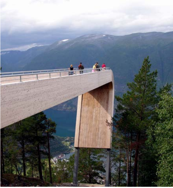
Glulam viewing bridge in Stegastein, on Aurlandsvegen, Norway.
