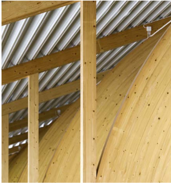
Glulam frame in cowshed.
