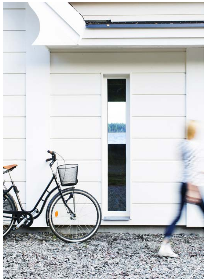
Glulam exterior cladding on façade.
