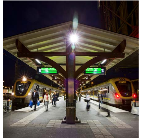
Platform roof, Gothenburg Central Station.
