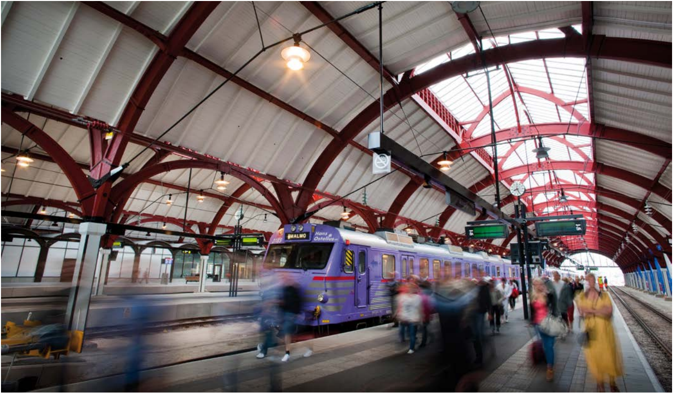
Malmö Central Railway Station main hall, built in 1923. This is one of the first great deliveries of glulam in Sweden. The station building is today in working order.
