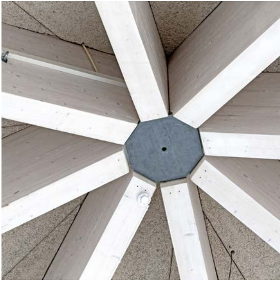
Detail of connection point in ridge.
