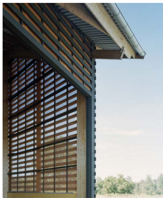
Barn with glulam load-bearing structure.
