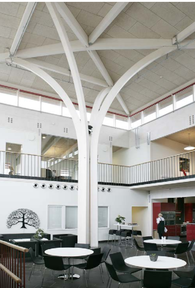
Glulam in an office environment.
