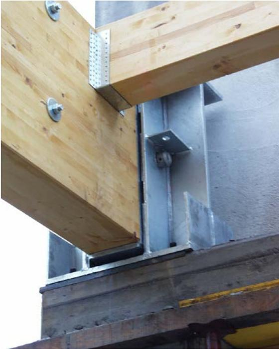
**Figure 16.16** Protection of end-pin-support by means of asbestos-free calcium silicate plates
