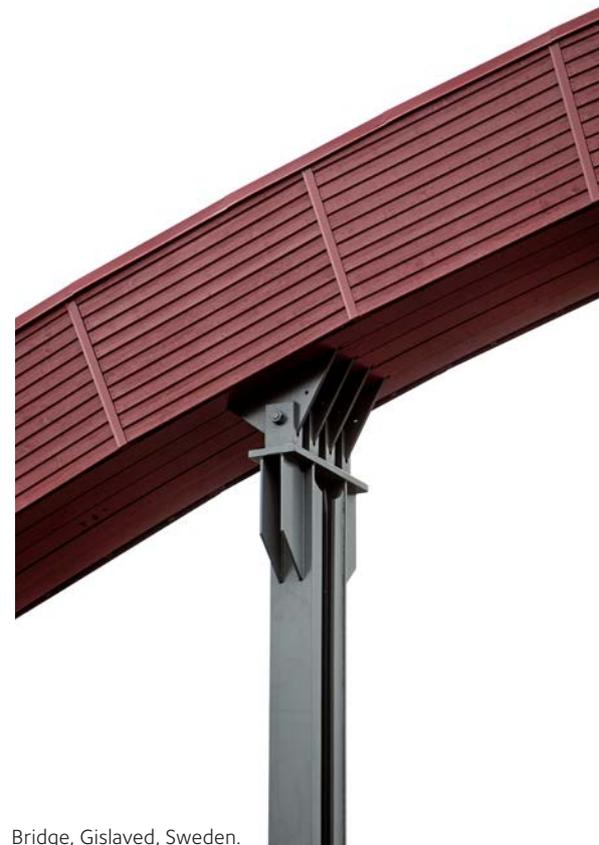
The wood is weakest in tension perpendicular to the grain, and such loading modes should in general be avoided. The figures below show a few situations where tension perpendicular to the grain will arise. A situation where there is an obvious risk of splitting failure due to tension perpendicular to the grain is when a beam is loaded by a connector as indicated in figure 14.5.
