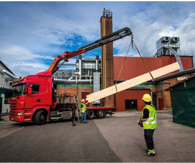
Using a crane to unload glulam elements from a truck.
