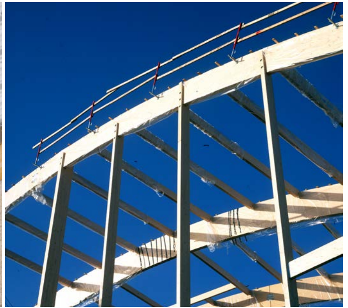
Glulam arches with glulam gable posts and purlins.
