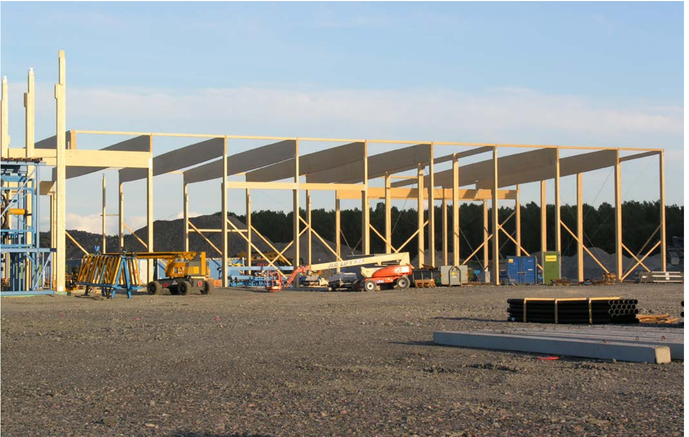
Glulam frame for industrial building under construction.
