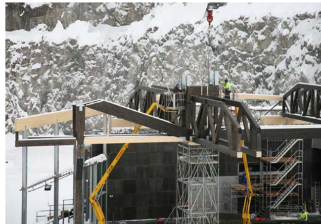
Assembling the glulam frame in the winter months without weather protection.
