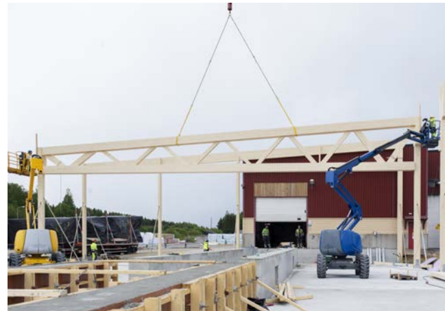
Assembling the glulam frame in the summer months without weather protection.
