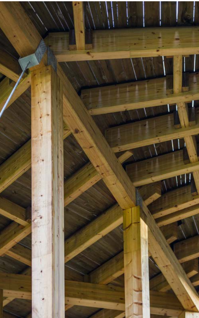
Fork bracket in wind brace for a glulam frame.
