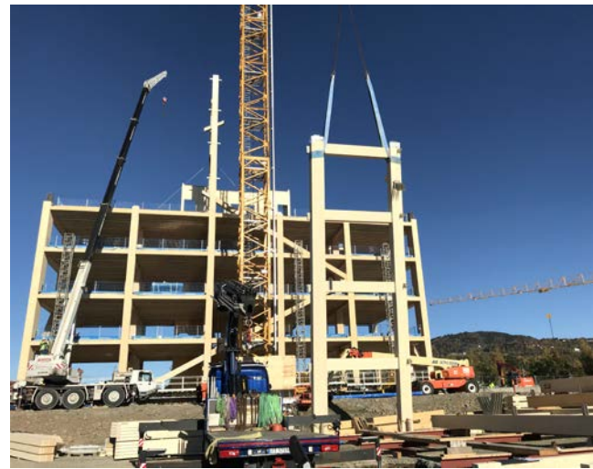
Assembling the glulam frame for a multi-storey building without weather protection.
