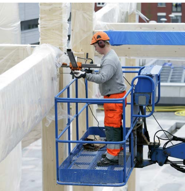
Assembling the glulam frame with original packaging as weather protection.
