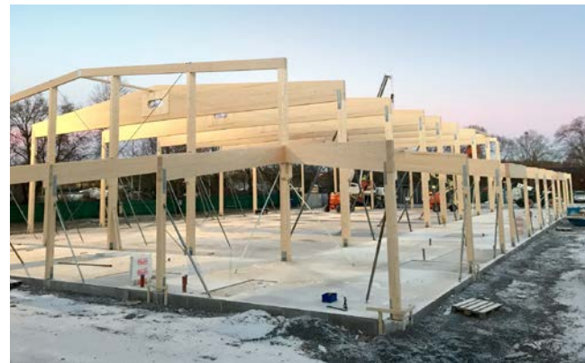
Temporary bracing when installing glulam frames.
