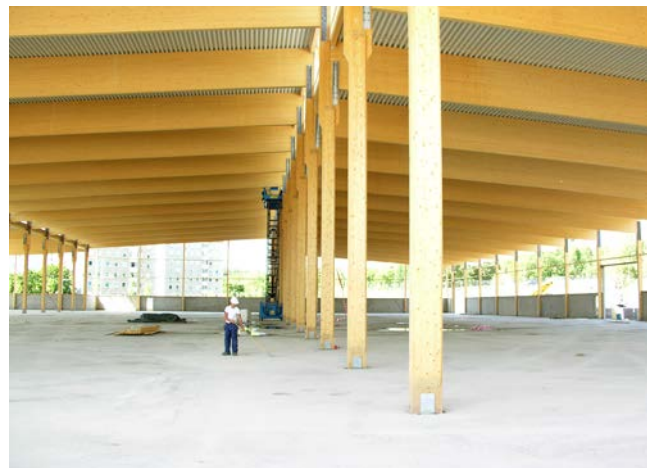
Completed glulam post and beam frame. Timber and builders' merchant.
