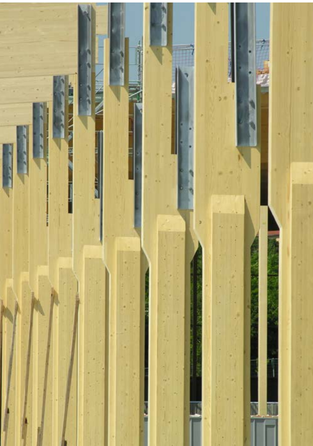
Assembled glulam posts with UPE profile plates at the top.
