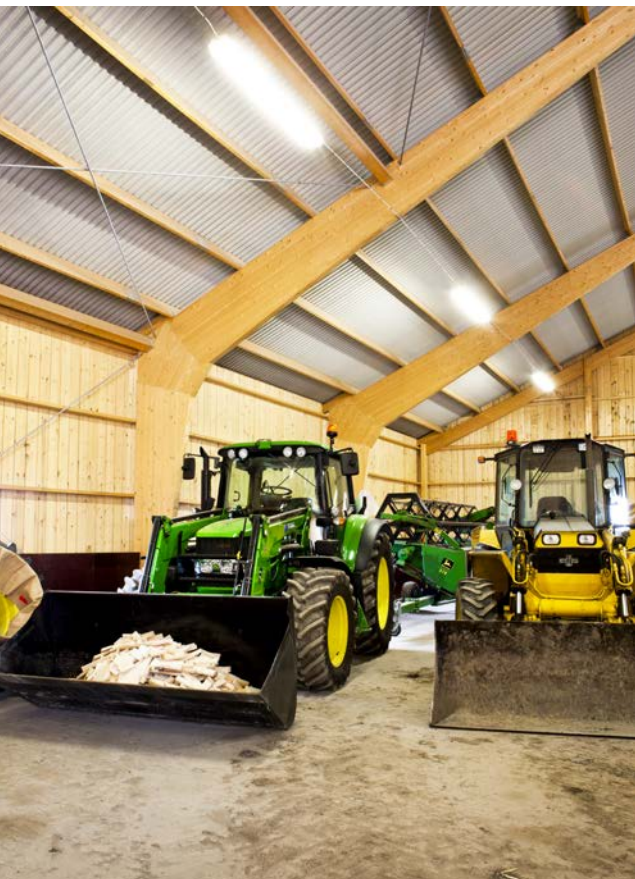
Permanent wind braces in completed machine hall with glulam frame.
