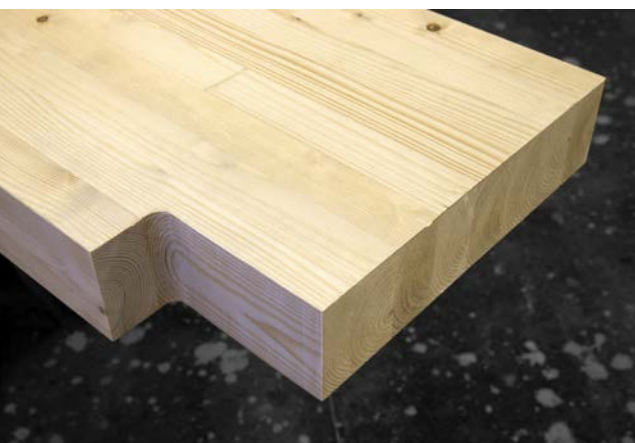
Notches without reinforcement are best made with a rounded inner corner.
