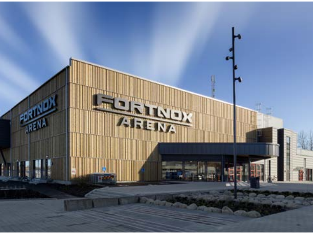
Floorball arena with glulam frame.
