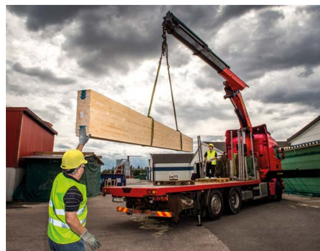
Truck unloading glulam delivery by crane.
