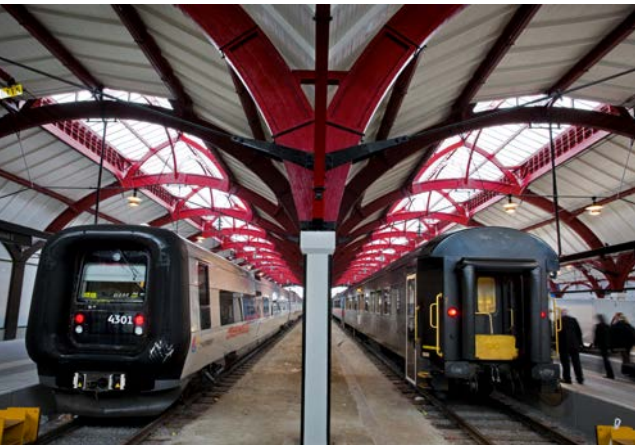
Malmö Central Station. Railway hall built in 1923. One of the first large deliveries of glulam in Sweden. The glulam is painted. The hall is still in use today.
