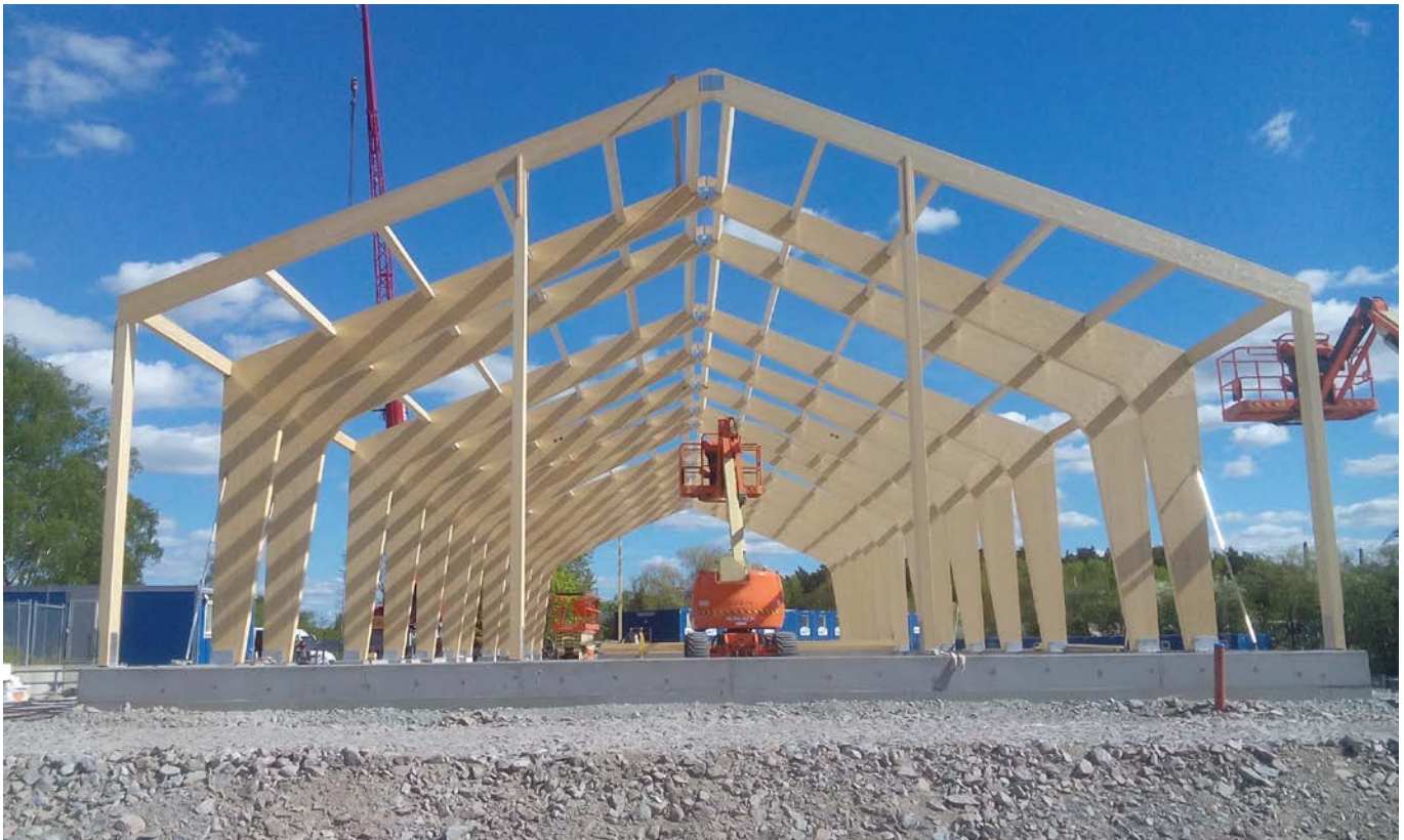
Completed frame of glulam portals with finger-jointed portal haunches. Warehouse.
