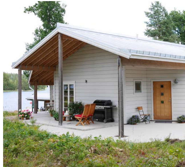
Holiday home with walls of painted glulam cladding. The glulam ridge beam and binders are partially exposed to the outdoors but protected under the roof.
