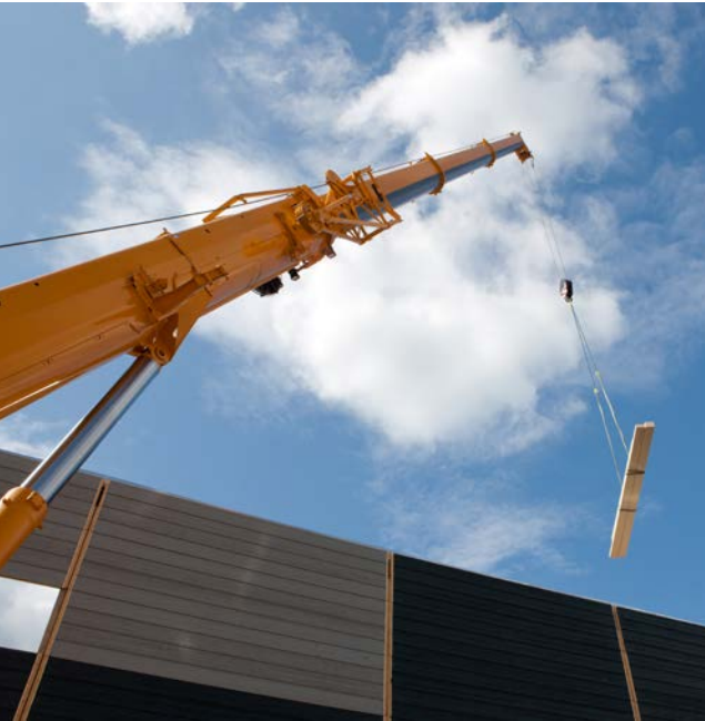
Lifting glulam elements with a mobile crane.
