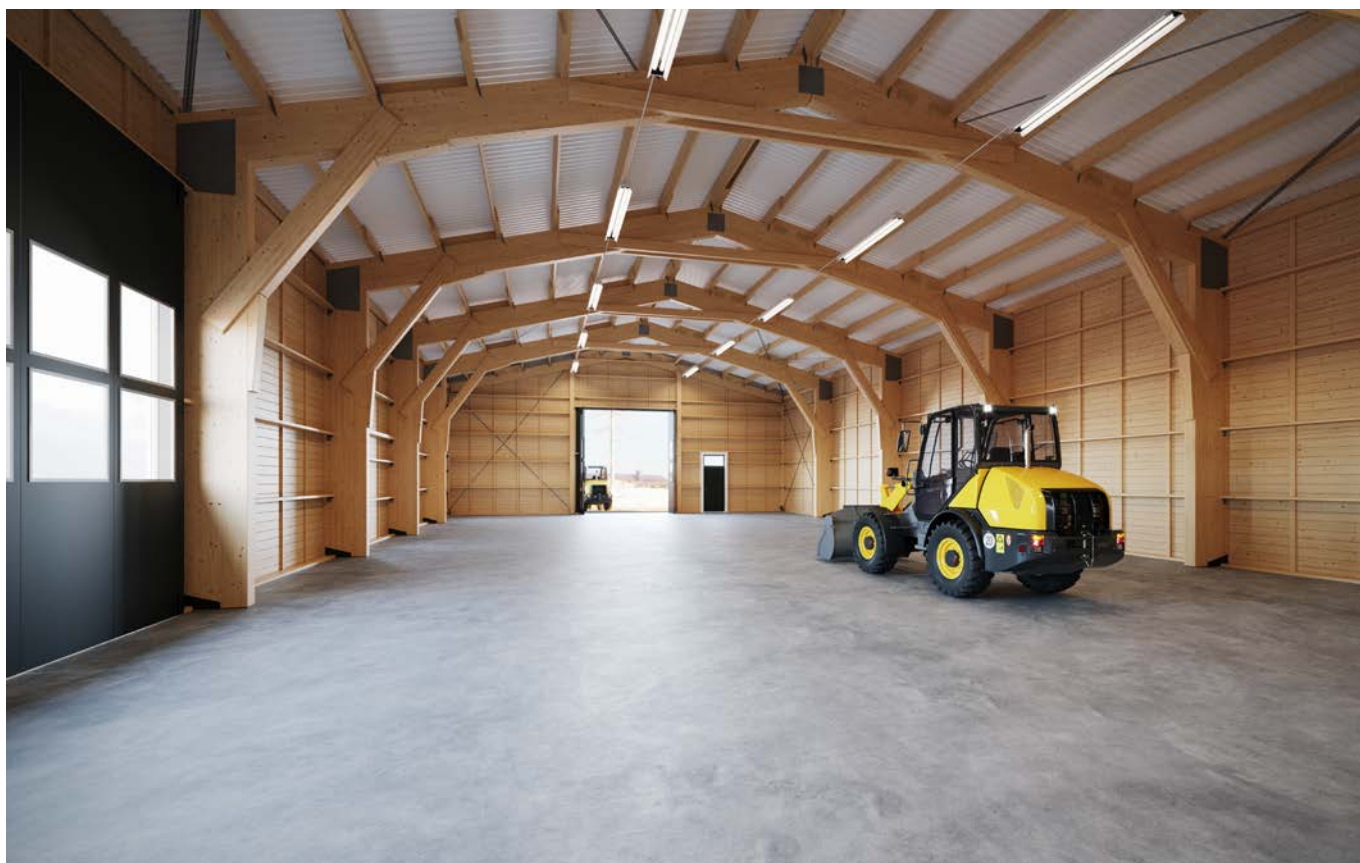
Machine hall with glulam frame.
